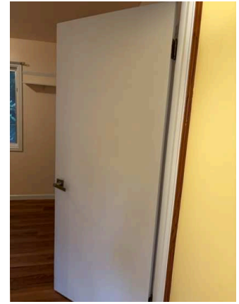
Interior Doors - Both Sides (16/21) 02/02/2026 11:12 AM
