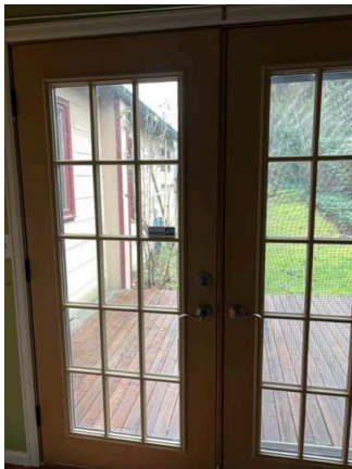
Exterior Doors - Both Sides (8/10) 02/02/2026 11:19 AM
