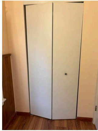
Interior Doors - Both Sides (15/21) 02/02/2026 11:11 AM
