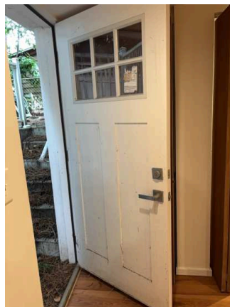
Exterior Doors - Both Sides (2/10) 02/02/2026 10:40 AM
