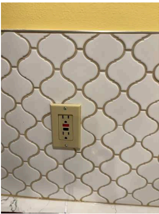
Switches / Outlets / Wall Plates (29/35) 02/02/2026 10:57 AM
