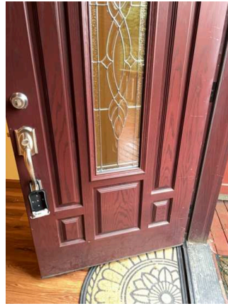
Exterior Doors - Both Sides (6/10) 02/02/2026 11:12 AM
