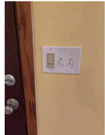
Switches / Outlets / Wall Plates (8/35) 02/02/2026 10:55 AM
