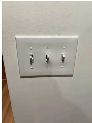
Switches / Outlets / Wall Plates (7/35) 02/02/2026 10:43 AM
