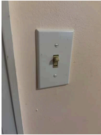
Switches / Outlets / Wall Plates (18/35) 02/02/2026 10:56 AM
