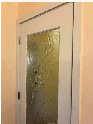
Interior Doors - Both Sides (9/21) 02/02/2026 11:11 AM
