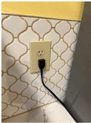
Switches / Outlets / Wall Plates (31/35) 02/02/2026 10:57 AM
