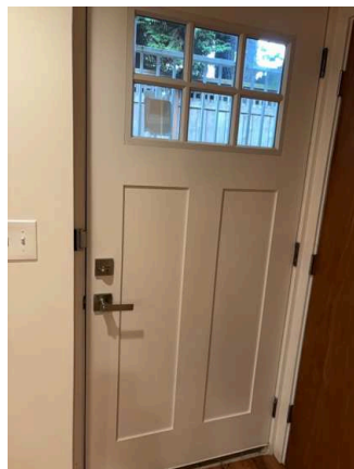
Exterior Doors - Both Sides (1/10) 02/02/2026 10:40 AM
