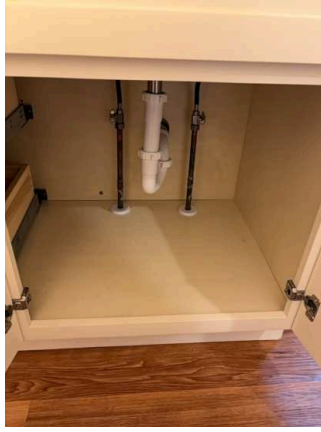
Under Bath Sink (2/6) 02/02/2026 11:16 AM
