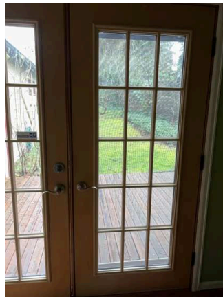
Exterior Doors - Both Sides (9/10) 02/02/2026 11:19 AM
