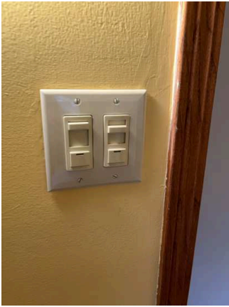
Switches / Outlets / Wall Plates (17/35) 02/02/2026 10:56 AM
