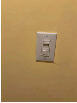
Switches / Outlets / Wall Plates (26/35) 02/02/2026 10:57 AM
