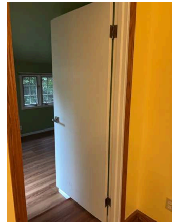
Interior Doors - Both Sides (20/21) 02/02/2026 11:12 AM
