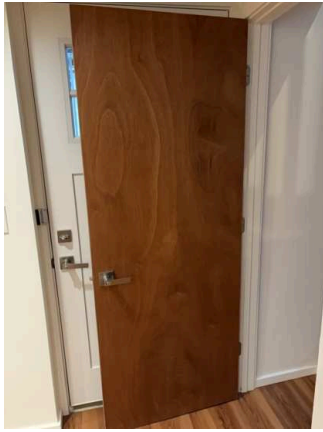
Interior Doors - Both Sides (1/21) 02/02/2026 10:39 AM
