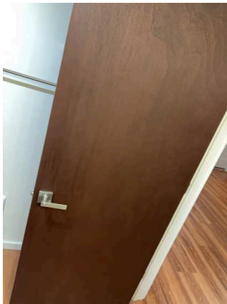
Interior Doors - Both Sides (5/21) 02/02/2026 10:40 AM
