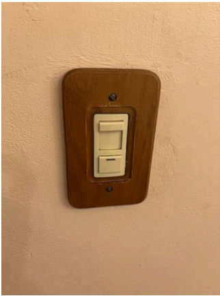
Switches / Outlets / Wall Plates (33/35) 02/02/2026 10:57 AM
