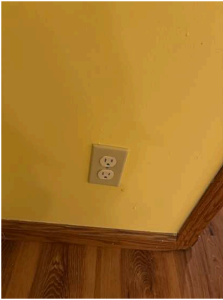
Switches / Outlets / Wall Plates (21/35) 02/02/2026 10:56 AM
