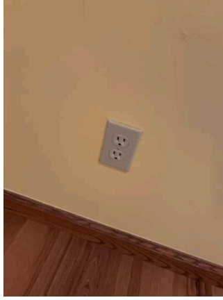
Switches / Outlets / Wall Plates (15/35) 02/02/2026 10:56 AM
