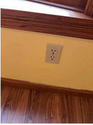
Switches / Outlets / Wall Plates (13/35) 02/02/2026 10:55 AM
