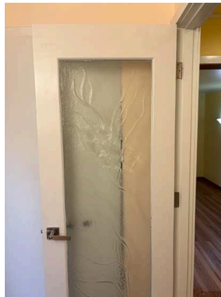
Interior Doors - Both Sides (7/21) 02/02/2026 11:11 AM
