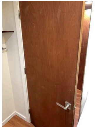
Interior Doors - Both Sides (6/21) 02/02/2026 10:40 AM
