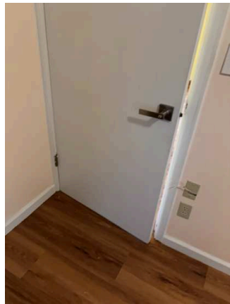
Interior Doors - Both Sides (18/21) 02/02/2026 11:12 AM
