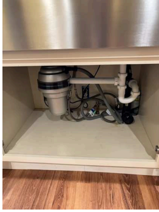
Under Kitchen Sink 02/02/2026 11:07 AM
