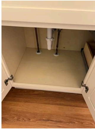
Under Bath Sink (6/6) 02/02/2026 11:16 AM
