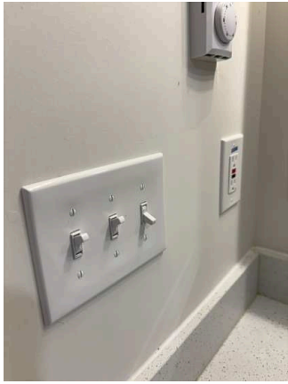
Switches / Outlets / Wall Plates (1/35) 02/02/2026 10:43 AM
