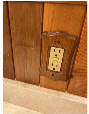
Switches / Outlets / Wall Plates (32/35) 02/02/2026 10:57 AM
