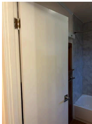
Interior Doors - Both Sides (11/21) 02/02/2026 11:11 AM
