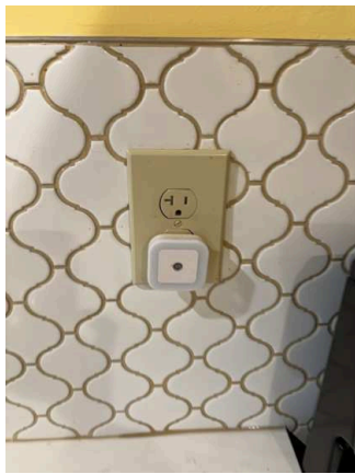
Switches / Outlets / Wall Plates (30/35) 02/02/2026 10:57 AM
