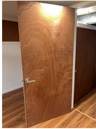
Interior Doors - Both Sides (3/21) 02/02/2026 10:39 AM
