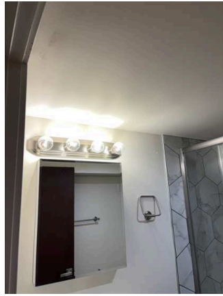
Light fixtures (3/21) 02/02/2026 10:43 AM
