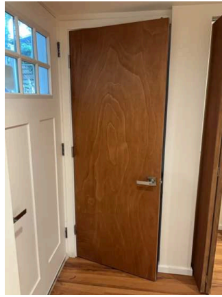
Interior Doors - Both Sides (2/21) 02/02/2026 10:39 AM
