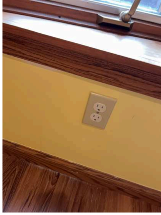
Switches / Outlets / Wall Plates (14/35) 02/02/2026 10:55 AM
