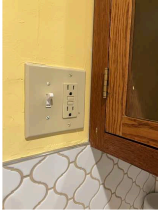
Switches / Outlets / Wall Plates (27/35) 02/02/2026 10:57 AM
