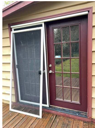
Exterior Doors - Both Sides (10/10) 02/02/2026 11:19 AM
