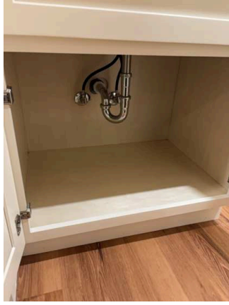
Under Bath Sink (1/6) 02/02/2026 10:46 AM
