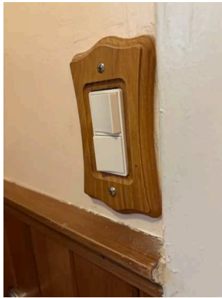
Switches / Outlets / Wall Plates (35/35) 02/02/2026 10:57 AM
