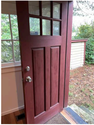
Exterior Doors - Both Sides (4/10) 02/02/2026 10:52 AM
