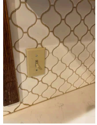
Switches / Outlets / Wall Plates (28/35) 02/02/2026 10:57 AM
