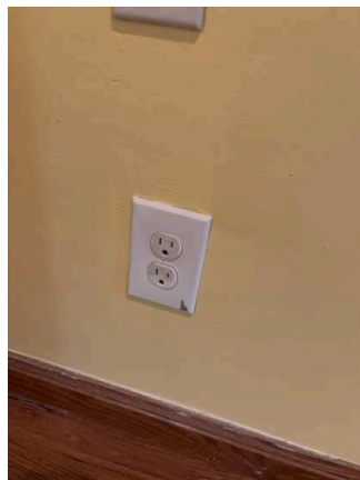
Switches / Outlets / Wall Plates (10/35) 02/02/2026 10:55 AM
