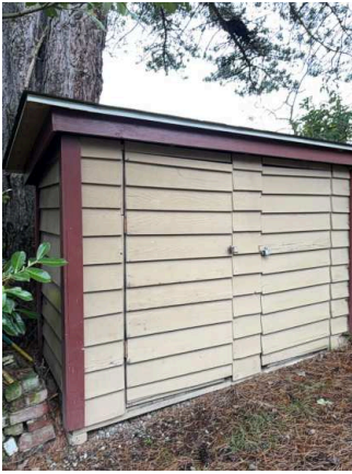
Shed / Outbuildings 02/02/2026 11:21 AM
