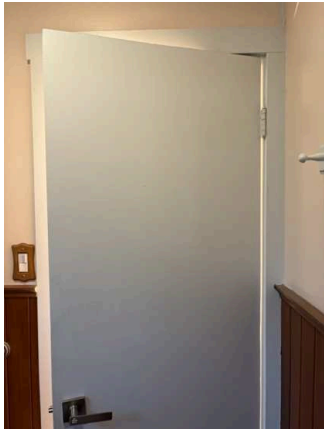
Interior Doors - Both Sides (13/21) 02/02/2026 11:11 AM
