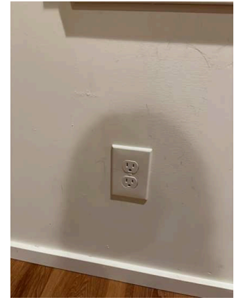
Switches / Outlets / Wall Plates (4/35) 02/02/2026 10:43 AM
