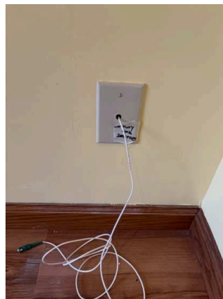
Switches / Outlets / Wall Plates (11/35) 02/02/2026 10:55 AM
