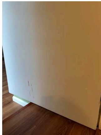
Interior Doors - Both Sides (19/21) 02/02/2026 11:12 AM
