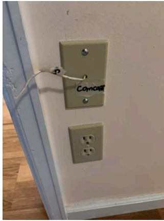
Switches / Outlets / Wall Plates (19/35) 02/02/2026 10:56 AM
