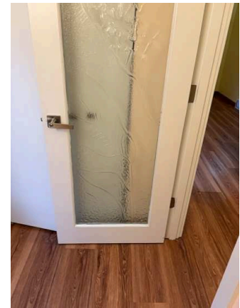
Interior Doors - Both Sides (8/21) 02/02/2026 11:11 AM
