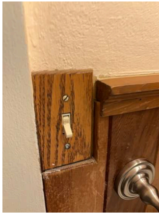
Switches / Outlets / Wall Plates (34/35) 02/02/2026 10:57 AM
