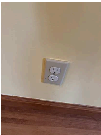
Switches / Outlets / Wall Plates (9/35) 02/02/2026 10:55 AM
