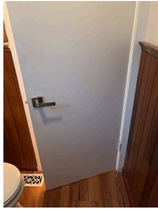
Interior Doors - Both Sides (14/21) 02/02/2026 11:11 AM
