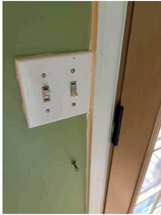
Switches / Outlets / Wall Plates (22/35) 02/02/2026 10:56 AM
