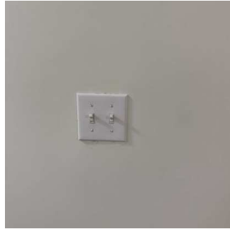
Switches / Outlets / Wall Plates (10/16) 01/15/2026 9:51 AM
