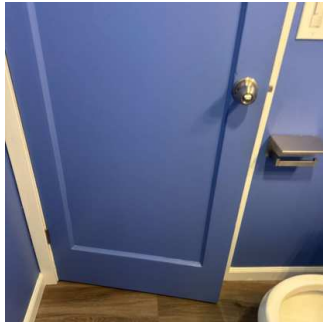
Interior doors continued (7/7) 01/15/2026 9:49 AM
