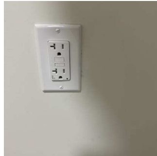
Switches / Outlets / Wall Plates (15/16) 01/15/2026 9:51 AM
