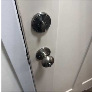
Pic of Front Door Lock (1/2) 01/15/2026 9:46 AM
