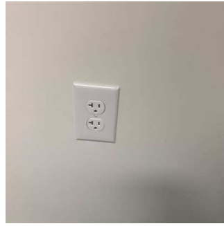
Switches / Outlets / Wall Plates (7/16) 01/15/2026 9:51 AM
