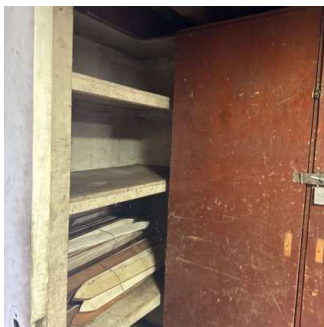
Shelving / Flooring (3/4) 01/15/2026 10:36 AM
