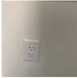
Switches / Outlets / Wall Plates (6/16) 01/15/2026 9:51 AM
