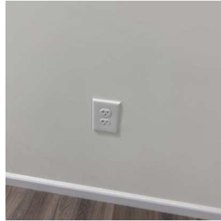
Switches / Outlets / Wall Plates (11/16) 01/15/2026 9:51 AM
