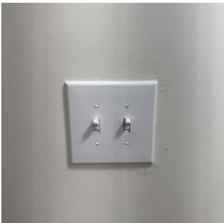
Switches / Outlets / Wall Plates (1/16) 01/15/2026 9:51 AM
