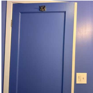
Interior doors continued (6/7) 01/15/2026 9:49 AM
