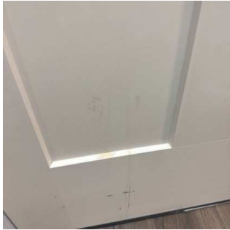
Exterior Doors - Both Sides (10/10) 01/15/2026 9:46 AM
