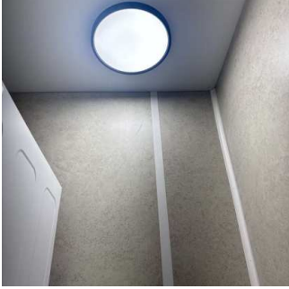
Light fixtures (4/10) 01/15/2026 9:56 AM
