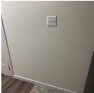
Wall continued (6/9) 01/15/2026 9:40 AM
