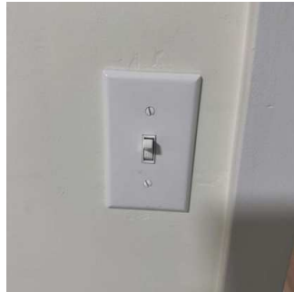
Switches / Outlets / Wall Plates (14/16) 01/15/2026 9:51 AM
