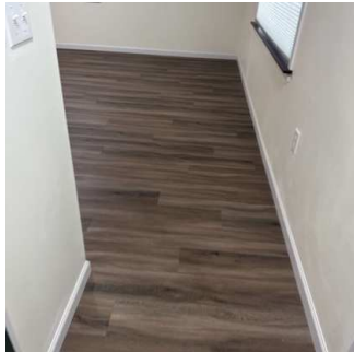
Laminate / Linoleum / Tile / Hardwoods (2/16) 01/15/2026 9:49 AM
