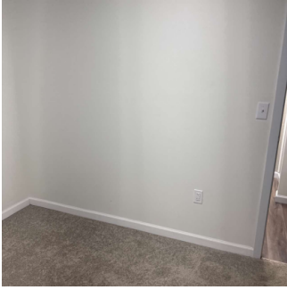
Walls continued (13/16) 01/15/2026 9:37 AM
