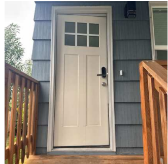
Exterior Doors - Both Sides (1/10) 01/15/2026 9:23 AM
