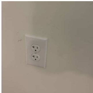
Switches / Outlets / Wall Plates (3/16) 01/15/2026 9:51 AM
