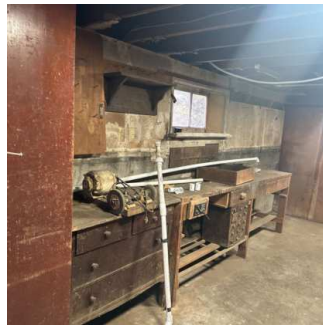
Shelving / Flooring (1/4) 01/15/2026 10:36 AM
