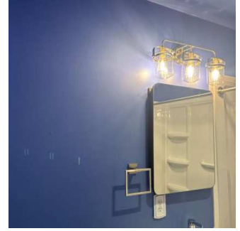
Walls continued 2 (16/16) 01/15/2026 9:39 AM
