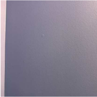
Walls continued 3 (1/16) 01/15/2026 9:39 AM
