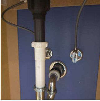
Under Bath Sink (2/5) 01/15/2026 10:22 AM
