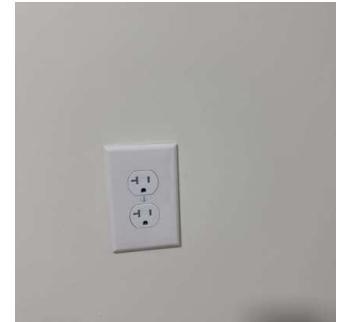
Switches / Outlets / Wall Plates (16/16) 01/15/2026 9:51 AM
