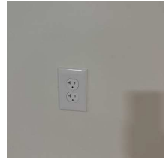
Switches / Outlets / Wall Plates (8/16) 01/15/2026 9:51 AM
