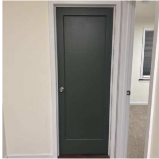
Interior doors continued (3/7) 01/15/2026 9:48 AM
