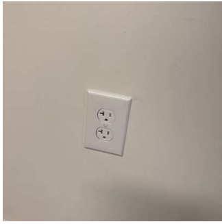
Switches / Outlets / Wall Plates (5/16) 01/15/2026 9:51 AM
