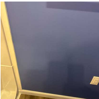
Walls continued 3 (9/16) 01/15/2026 9:39 AM
