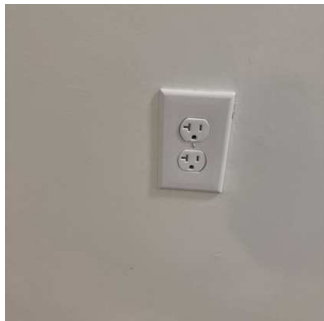
Switches / Outlets / Wall Plates (2/16) 01/15/2026 9:51 AM
