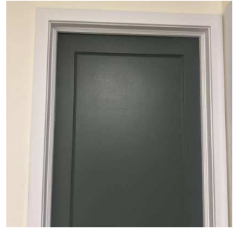
Interior doors continued (4/7) 01/15/2026 9:48 AM
