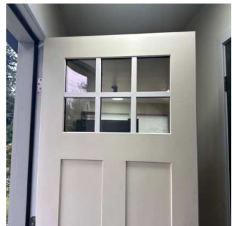
Exterior Doors - Both Sides (5/10) 01/15/2026 9:46 AM
