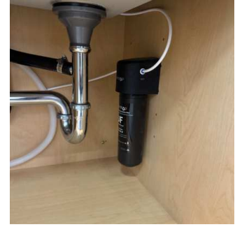
Under Kitchen Sink (2/2) 01/15/2026 10:04 AM
