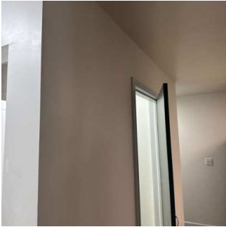
Walls continued 2 (1/16) 01/15/2026 9:38 AM
