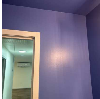
Walls continued 3 (2/16) 01/15/2026 9:39 AM
