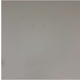
Walls continued (2/16) 01/15/2026 9:36 AM
