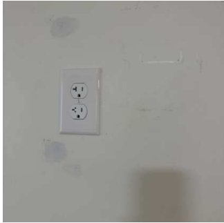
Switches / Outlets / Wall Plates (9/16) 01/15/2026 9:51 AM
