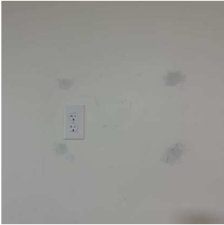
Walls continued (1/16) 01/15/2026 9:36 AM
