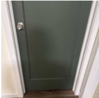
Interior doors continued (5/7) 01/15/2026 9:48 AM
