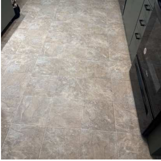
Laminate / Linoleum / Tile / Hardwoods (13/16) 01/15/2026 9:50 AM
