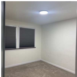
Walls continued (11/16) 01/15/2026 9:37 AM
