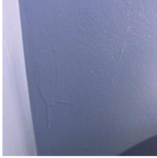
Walls continued 3 (14/16) 01/15/2026 9:39 AM
