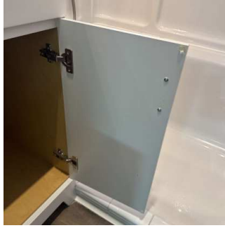
Under Bath Sink (4/5) 01/15/2026 10:22 AM
