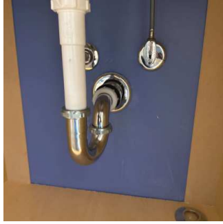
Under Bath Sink (3/5) 01/15/2026 10:22 AM
