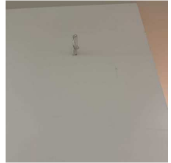
Walls continued (4/16) 01/15/2026 9:36 AM
