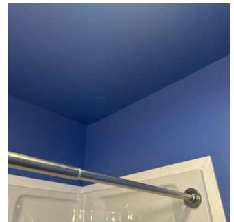
Walls continued 3 (12/16) 01/15/2026 9:39 AM
