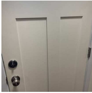
Exterior Doors - Both Sides (8/10) 01/15/2026 9:46 AM
