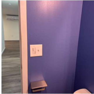
Walls continued 3 (3/16) 01/15/2026 9:39 AM
