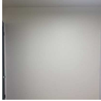
Walls continued (14/16) 01/15/2026 9:37 AM
