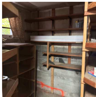
Shelving / Flooring (4/4) 01/15/2026 10:36 AM
