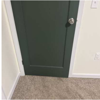
Interior doors continued (2/7) 01/15/2026 9:48 AM
