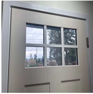
Exterior Doors - Both Sides (7/10) 01/15/2026 9:46 AM
