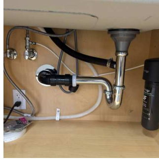
Under Kitchen Sink (1/2) 01/15/2026 10:04 AM
