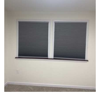
Walls continued (16/16) 01/15/2026 9:37 AM
