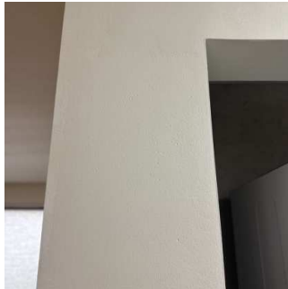
Walls continued (7/16) 01/15/2026 9:36 AM
