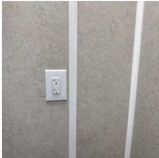
Switches / Outlets / Wall Plates (13/16) 01/15/2026 9:51 AM
