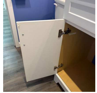
Under Bath Sink (5/5) 01/15/2026 10:22 AM
