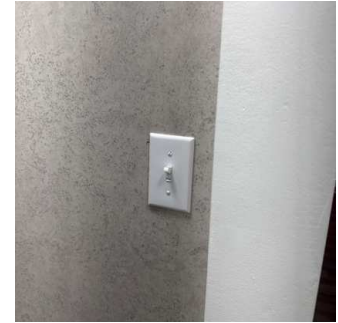
Switches / Outlets / Wall Plates (12/16) 01/15/2026 9:51 AM
