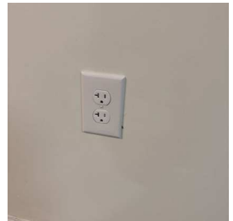
Switches / Outlets / Wall Plates (4/16) 01/15/2026 9:51 AM
