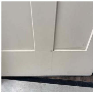
Exterior Doors - Both Sides (3/10) 01/15/2026 9:23 AM
