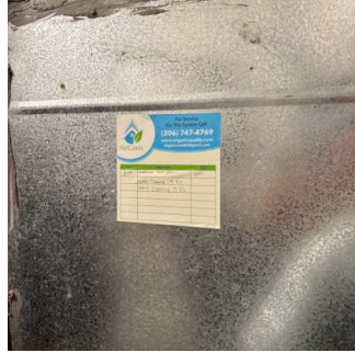
Has tenant replaced furnace filter? (Picture of filter + dimension) 09/18/2025 1:08 PM
